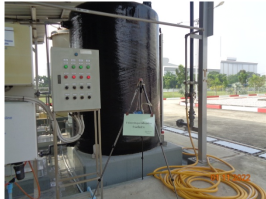
Chemical Feed Cooling Tower Block 2
